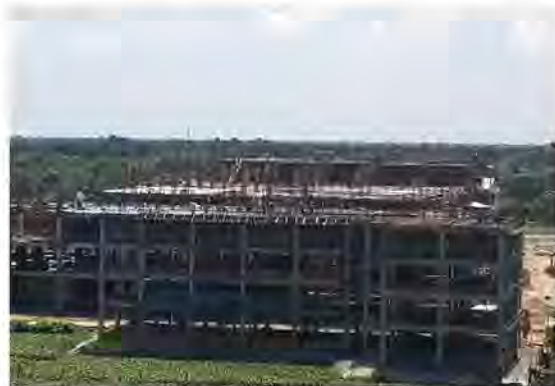
An underconstruction Green Factory of DIRD group financed by UCB
