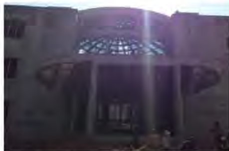
Project site of Imperial Hospital Limited finance by UCB
