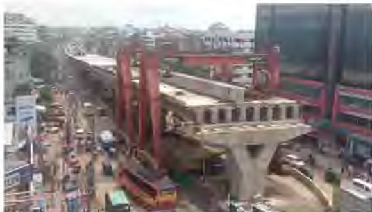
Construction of Muradpur Flyover, Chittagong, is under process
